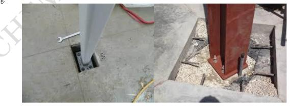
**CHEMfix Grout** may be placed in thicknesses from 10mm up to 100mm in a single pour when used as general grouting. Grout bolt holes and pockets prior to grouting between the substrate and base plate. Chains or metal straps laid in the formwork prior to placing may be necessary to assist grout flow. Pour the grout continuously from one side of the void to
